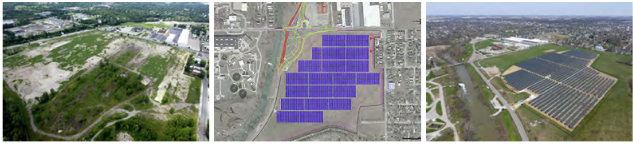
Solar facilities at the Continental Steel site: from contaminated land to an energy-producing community asset. (Source: Kokomo Tribune and IDEM)
