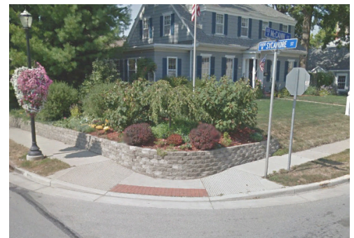
Figure 14.4 - This parallel and diagonal curb ramp can be found at the intersection of Sycamore and McCann Streets.
