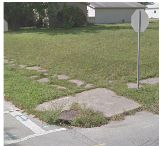
Figure 17.2 - This sidewalk and curb ramp is another example of non-compliant grade changes due to poor surface condition.
