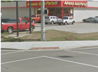
Figure 14.1 - This blended transition found at Apperson Way and Markland Avenue is also a diagonal curb ramp
