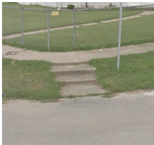
Figure 17.1 - These steps leading into the street at Lafayette Circle and Columbus Boulevard is an extreme case of non-compliant grade changes.
