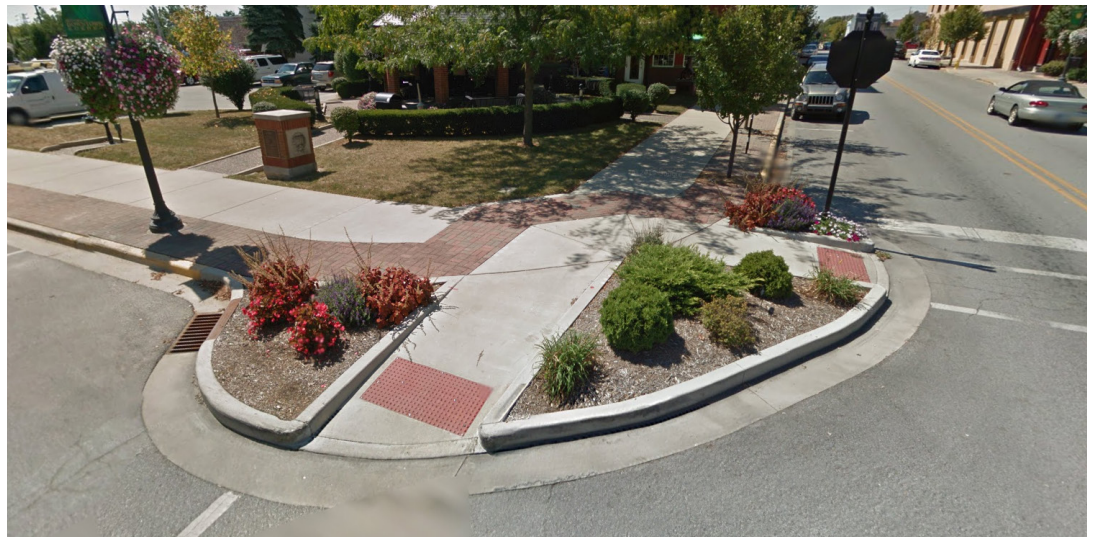
Figure 13.1 - This corner of Sycamore and Union Streets illustrates an adequate amount of space needed for a landing, passing, or turning (the clear space at the top of both curb ramps).
