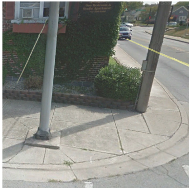
Figure 12.2 - These traffic signal and utility poles at the corner of Walnut and Philips Streets are good examples of a fixed obstruction.
