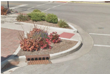
Figure 16.2 - Union and Sycamore Streets shows a proper technique to prevent drainage issues at the ramp.
