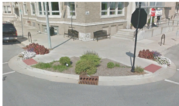
Figure 14.3 - Perpendicular curb ramp found at Union and Mulberry Streets.
