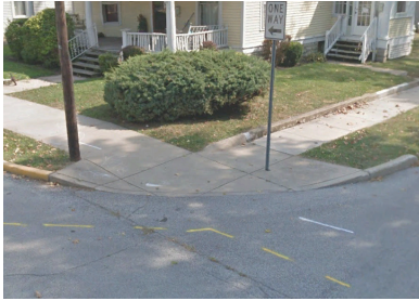
Figure 16.1 - Webster and Taylor Streets shows a lack of detectable warning devices.
