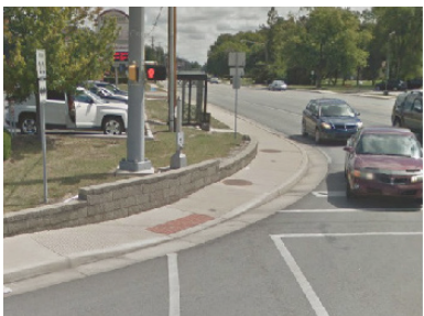
Figure 14.2 - Diagonal curb ramp found at Sycamore Street and Dixon Road.
