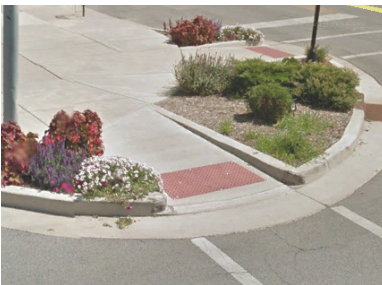
Figure 15.1 - The corner of Union and Mulberry Streets show a proper use of detectable warning.
