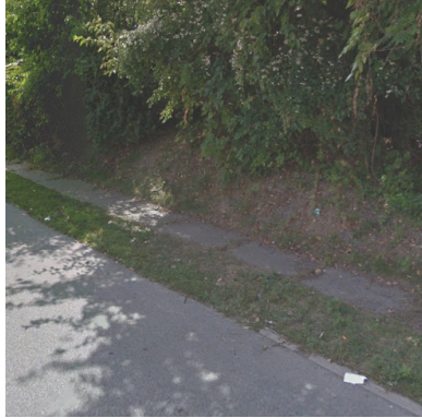
Figure 12.1 - Sidewalk found along Indiana Avenue with improper passing width.
