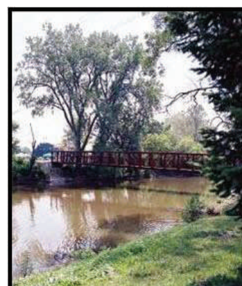
Foot bridge from Foster Park to Kokomo Beach.
